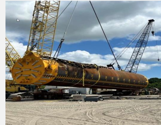
Mooring pile trial lift
