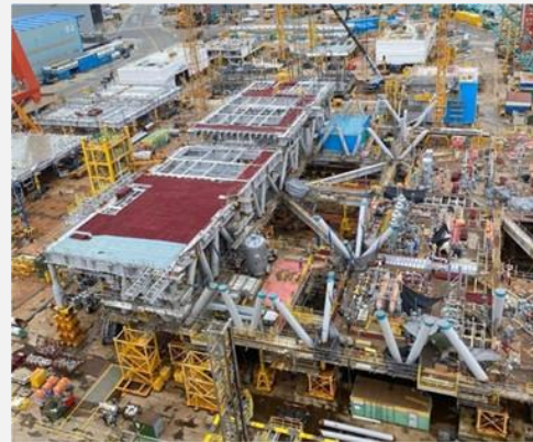
FPS – Stacking of Upper Deck on Lower Deck
